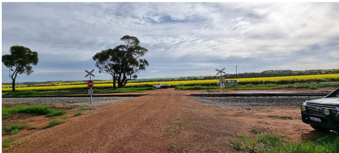
FIGURE 19. IMAGE OF THE UNPROTECTED LC NEAR YORK. IMAGE TAKEN FROM THE SPENCERS BROOK – YORK ROAD.
